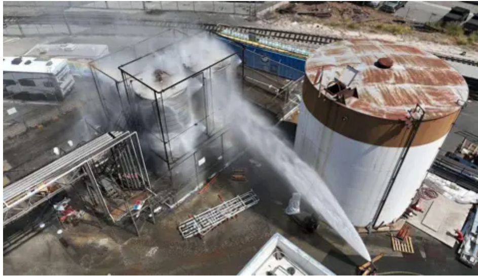
Figure 1: Firefighters Cooling Tank
