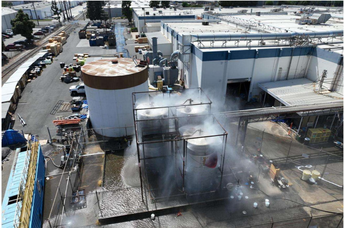
Figure 2. Aerial photograph of emergency cooling/suppression operations directed at storage tanks at the GKN Aerospace facility in Garden Grove. 3
